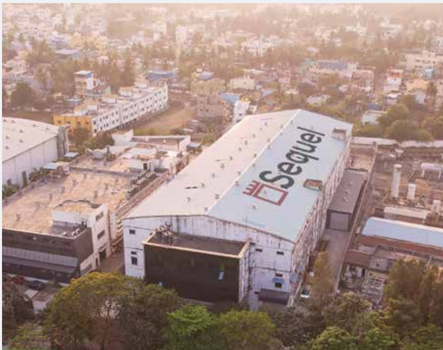
Sequel's bullion vaulting facility at MEPZ, Chennai
